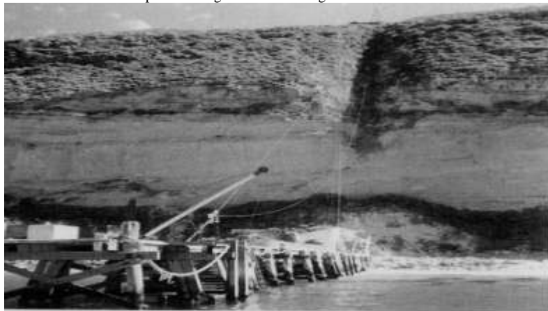
Althorp Island Jetty in 1972 showing a flying fox used for lifting cargo up to the island
