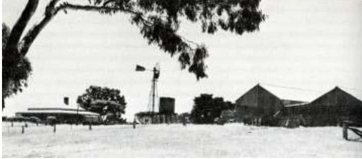
Inglewood homestead and outbuildings as purchased by the AMP Society
