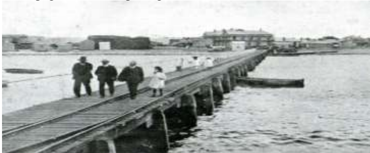
The old jetty at Tumby Bay
