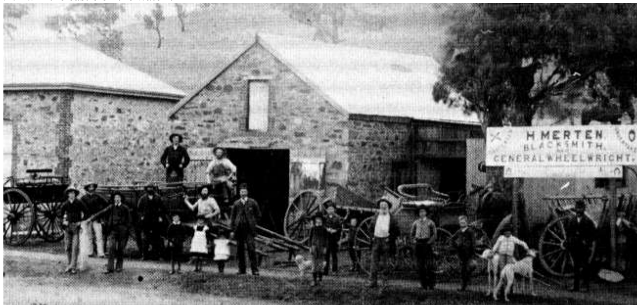
H. Merten's blacksmith's shop at Truro
