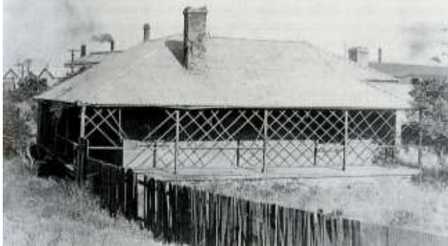
Colonel Light's Cottage – Demolished in 1926
