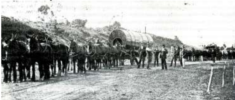
A boiler and other equipment bound for Tarcoola in 1900
