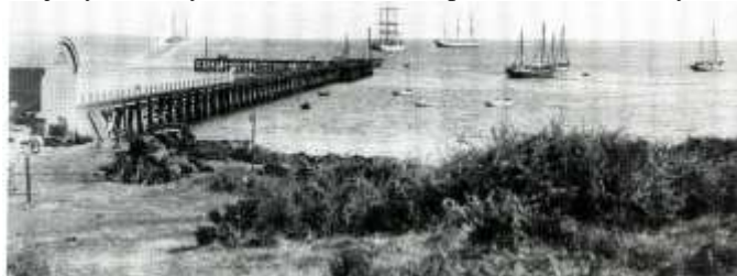
Port Victoria jetty - 1913
